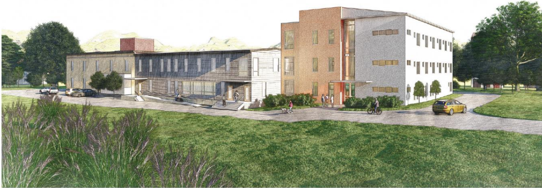
RENOVATED BUILDING WITH NEW ADDITION - VIEW OF NORTH FACADE LOOKING SOUTHEAST
